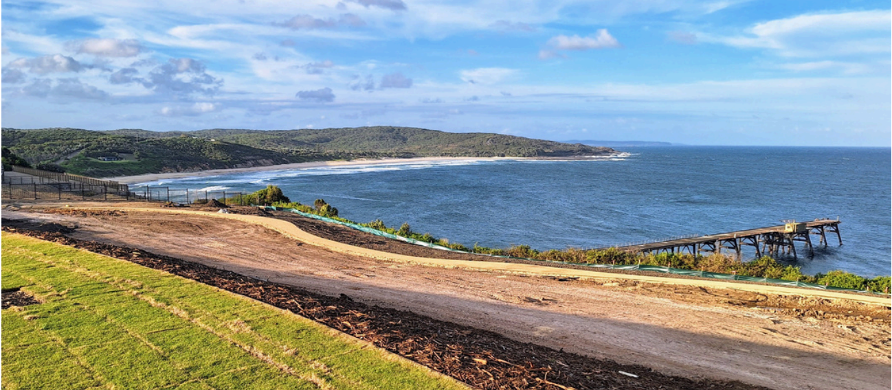
Catho Coastal Walkway under construction on the southern headland
