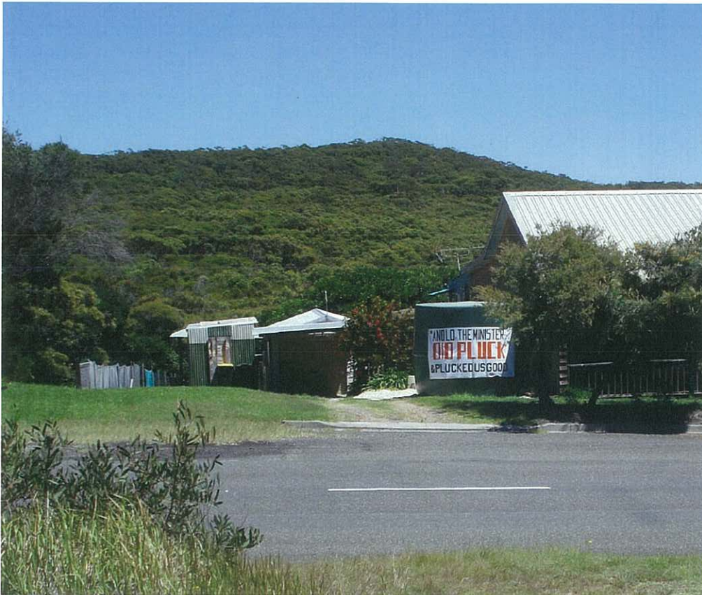
2. View of Area C from Flowers Drive. Bushland backdrop will be destroyed.
